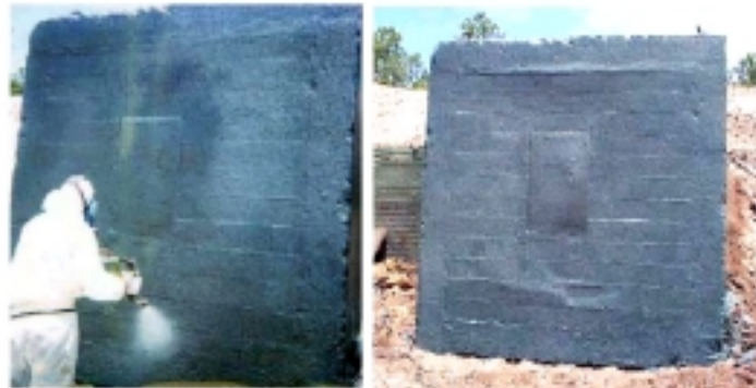
Spraying Polymer
